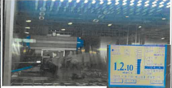
Leakage Stem Seal: 1.2 E-06
